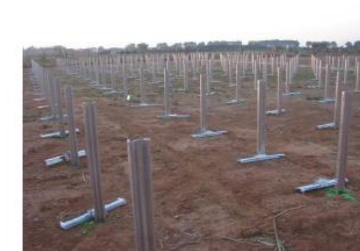
Aspect des supports
